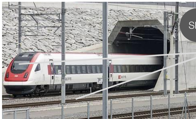
Points, Signals, On-Board Unit
